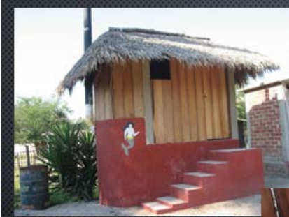
RILES Compost Toilet in Maruata, Michoacan, Mexico
